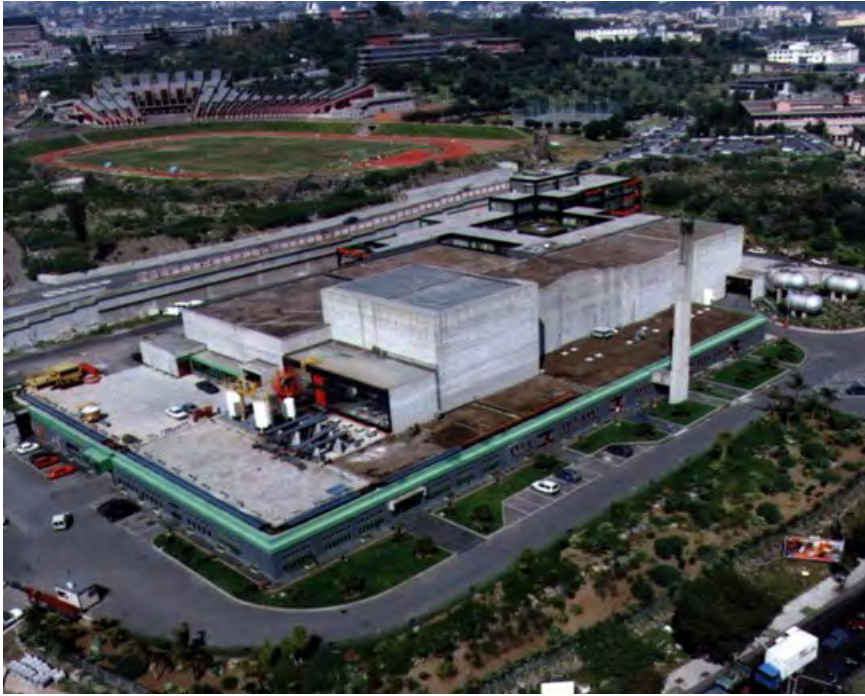
Figure 13.49: Aerial view of LNS.
