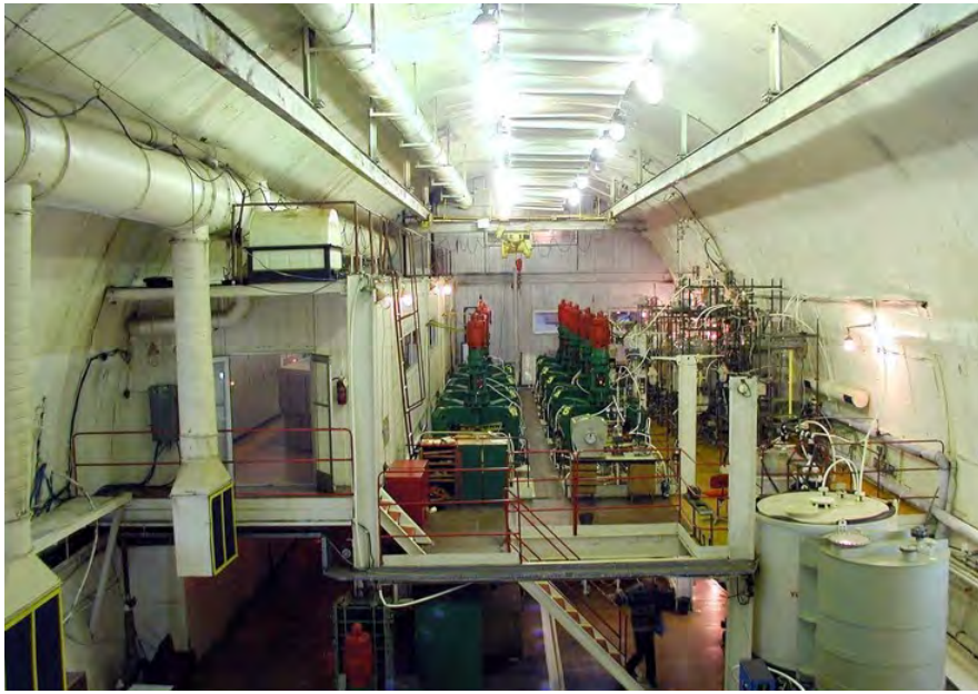
Figure 13.80: Irradiation facility for radioisotope production at 160-MeV proton beam of INR-linac.
