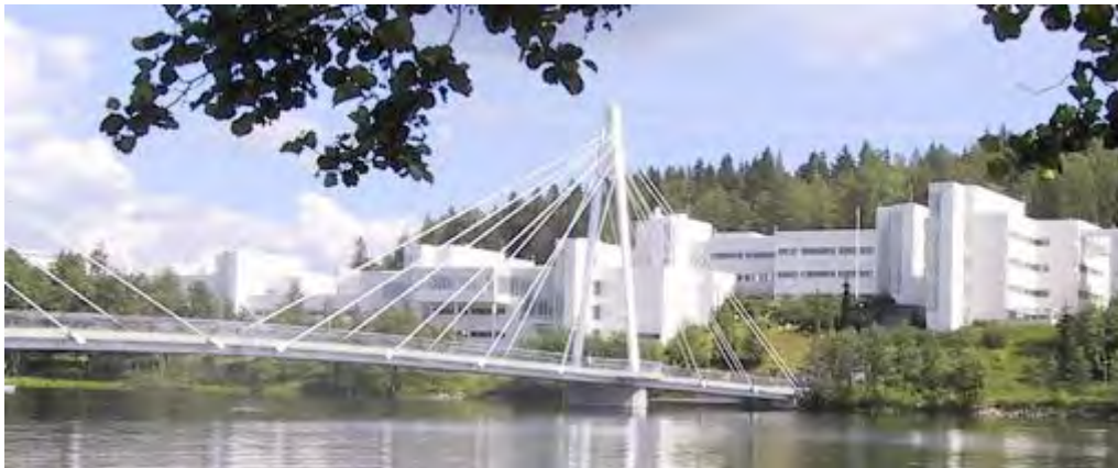
Figure 13.7: View of the Department of Physics at the Ylistö campus area.
