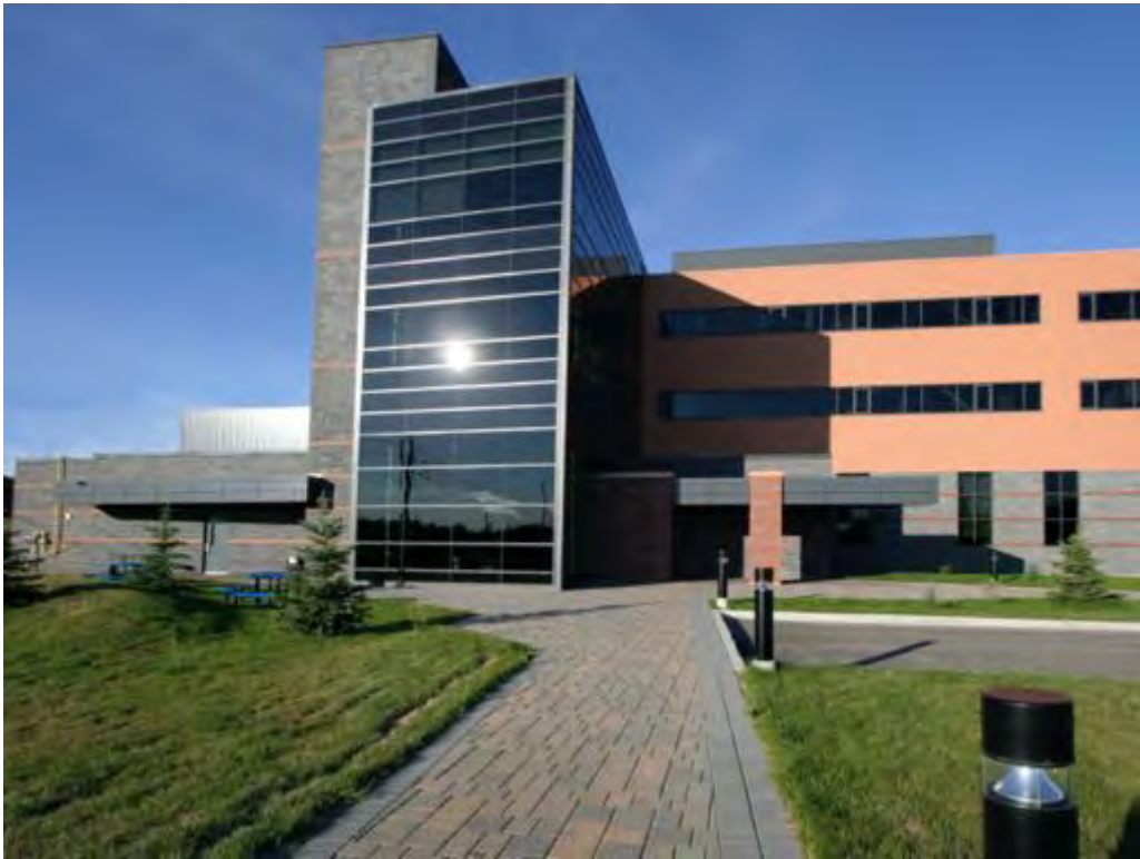
Figure 14.2: The surface building provides clean room space, change facilities, meeting rooms and office space for the underground experiments.
