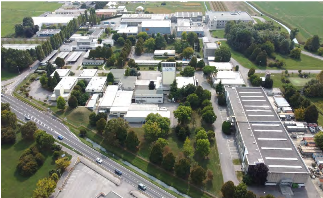
Figure 13.54: Aerial photo of the facility.
